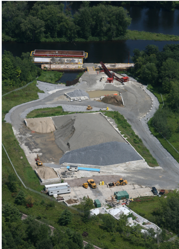
Moreau Backfill Loading Facility
